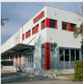
Logistics center in Leinfelden-Echterdingen
