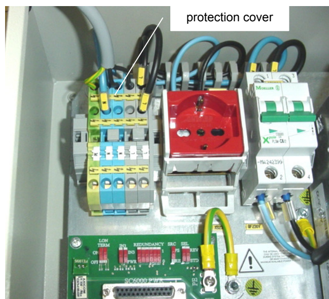
AC Line Terminal Block with Protection Covers
