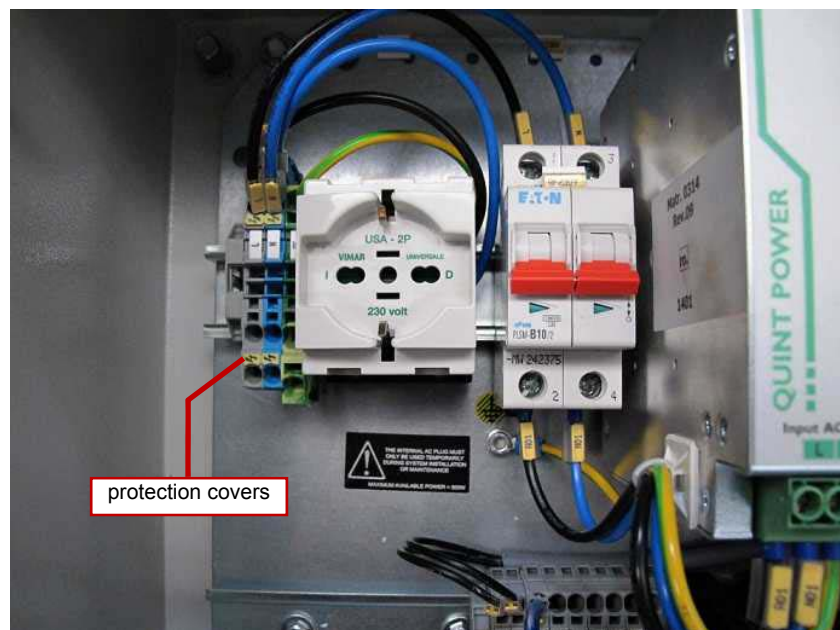
Figure 7 – PWR-480B AC Line Terminal Block with Protection Covers
